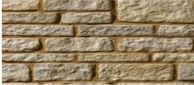
(iii) **Ashlar rock or quarry faced masonry:** In this type of ashlar masonry, a strip about 25mm wide and made by means of a chisel is provided around the perimeter of every stone exposed for view. But the remaining portion of the face is left in the same form as received from quarry. Only projections on the face known as bushings exceeding 80mm are removed by a hammer. This type of construction gives massive appearance.
