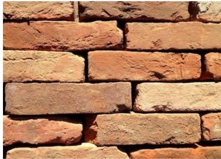
**(ii) Burnt Bricks:** The bricks used in construction works are burnt bricks and they are classified into the following four categories.
